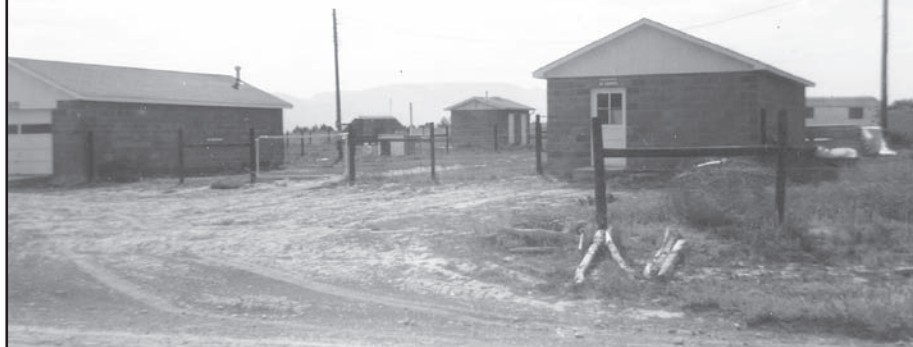
The Machine shop, left, Woodshop, right, and Mabel I house in the background, as they appeared in February 1963. Both shop buildings were expanded with additions later.
